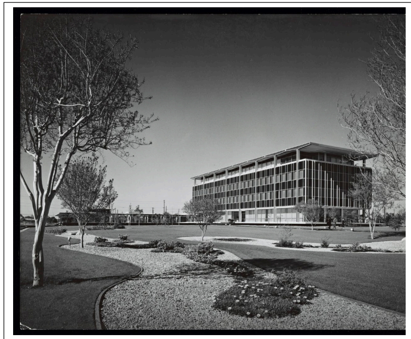
Headquarters building within landscaped setting 1962 photo by Jules Shulman
