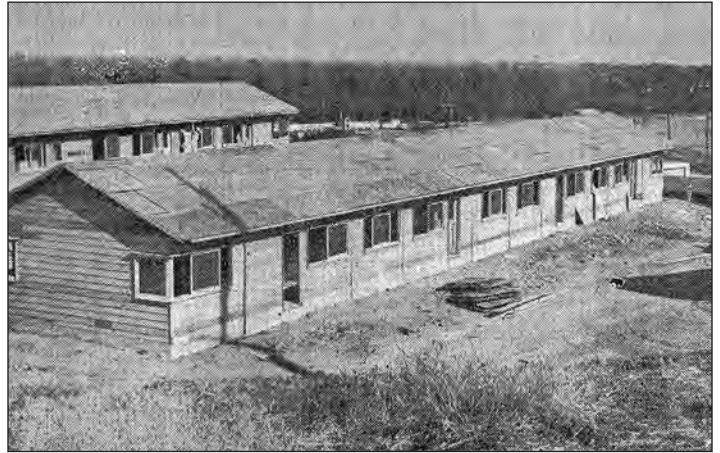
Veteran housing units being installed in 1946. The units remained on campus until 1955.
