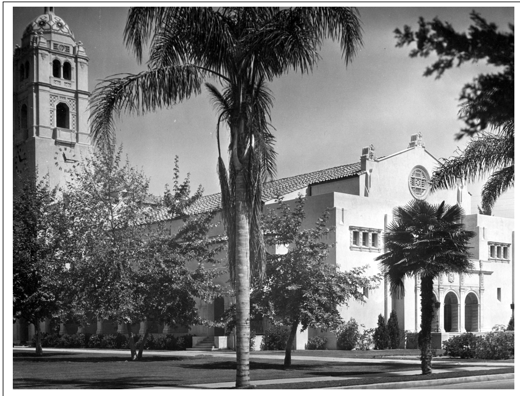
Fullerton Auditorium (formerly Plummer Auditorium), 1934
