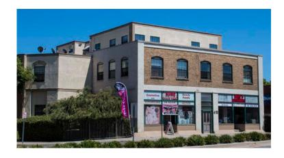
Constructed of un-reinforced masonry walls in 1923, this rectangular building was typical of many brick commercial structures of that era. The front façade has gold and tan wire-cut brick, framed in wide bands of cream-colored glazed brick. The second story features five identical double-hung windows, recessed in arched openings with projecting sills.
